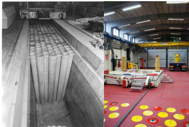
Figure 3: Waste storage facility, under construction (left) and nowadays (right)
